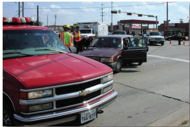
Figure 4.4. When the incident occurs in an intersection, it may be necessary to shield the work zone from multiple directions. Courtesy of Ron Moore, McKinney, TX, Fire Department.
